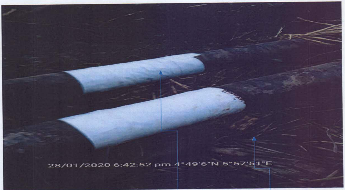
REPAIR POINT (WRAPPED)
